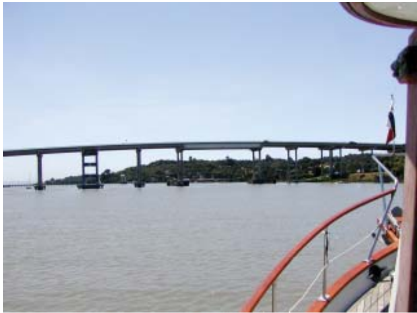
This fixed highway bridge limits Petaluma River traffic to 70' mast height.
